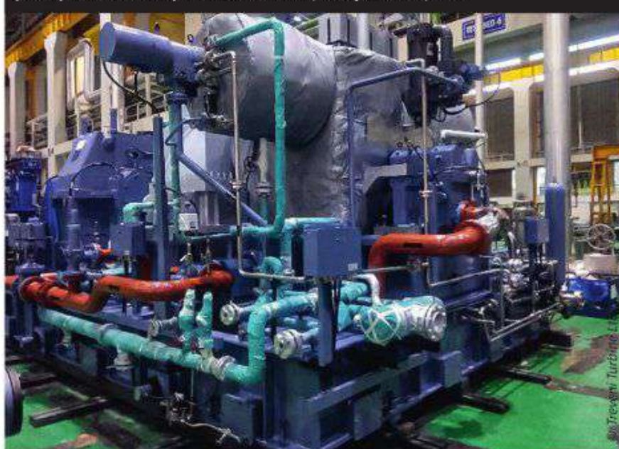
Triveni Turbines' 22 MW Injection Condensing Steam Turbine Generator (STG) for a WHR-based power plant in a cement plant located in Satna, Madhya Pradesh, India
