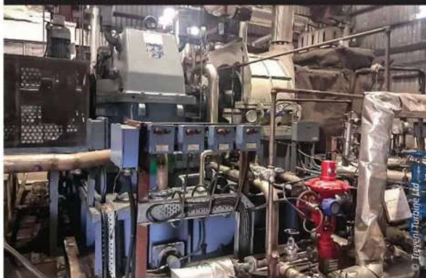
Steam turbine generator (STG) installed in a cement plant in India for generating power by sourcing waste heat from the process
