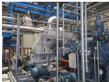
1. Waste-to-energy (WtE) power plants burn garbage to produce steam for use in turbines, such as the one shown here, to generate electricity and also to supply district heating systems in some communities. Courtesy: Triveni Turbines
