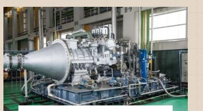
The project is driven by 1\*6.8 MWe Axial Exhaust Injection Condensing steam turbines with an inlet steam parameter of 15 Bar and 387 Deg C with 0.1 Bar Exhaust
