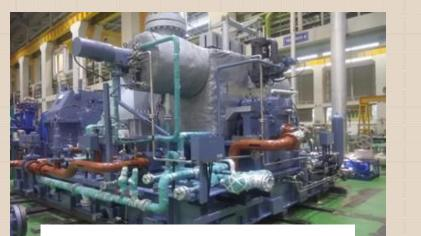
The project is driven by 1\*22.5 MWe Injection Condensing steam turbines with an inlet steam parameter of 12 Bar and 425 Deg C with 0.2 Bar Exhaust
