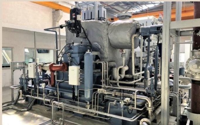
The project is driven by a 16 MW Condensing Steam Turbine with an inlet steam parameter of 42 Bar and 450 Deg C with 0.1 Bar Exhaust
